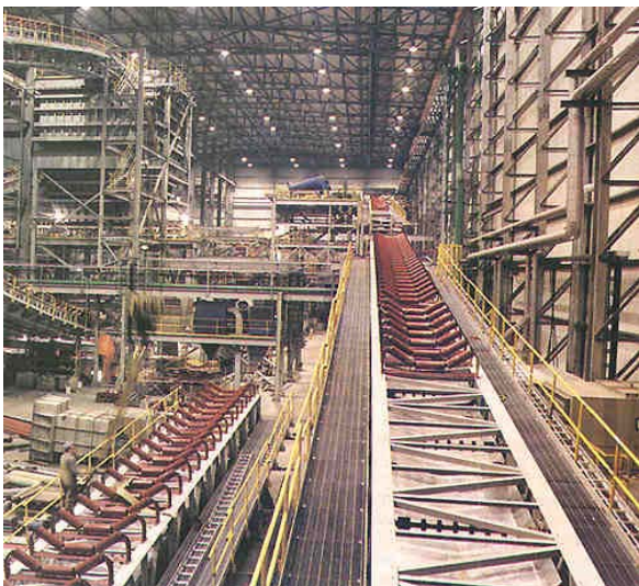
Inside view of Plant
